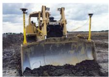
Parking lots always present a challenge to earthmoving contractors. Their irregular surfaces require extensive grade checking, and traditional rotating laser systems cannot be employed for machine control. Machine operators now skillfully grade these surfaces quickly and easily with the use of the Global Positioning System (GPS) for machine guidance, one of the most innovative areas of today's construction industry.
